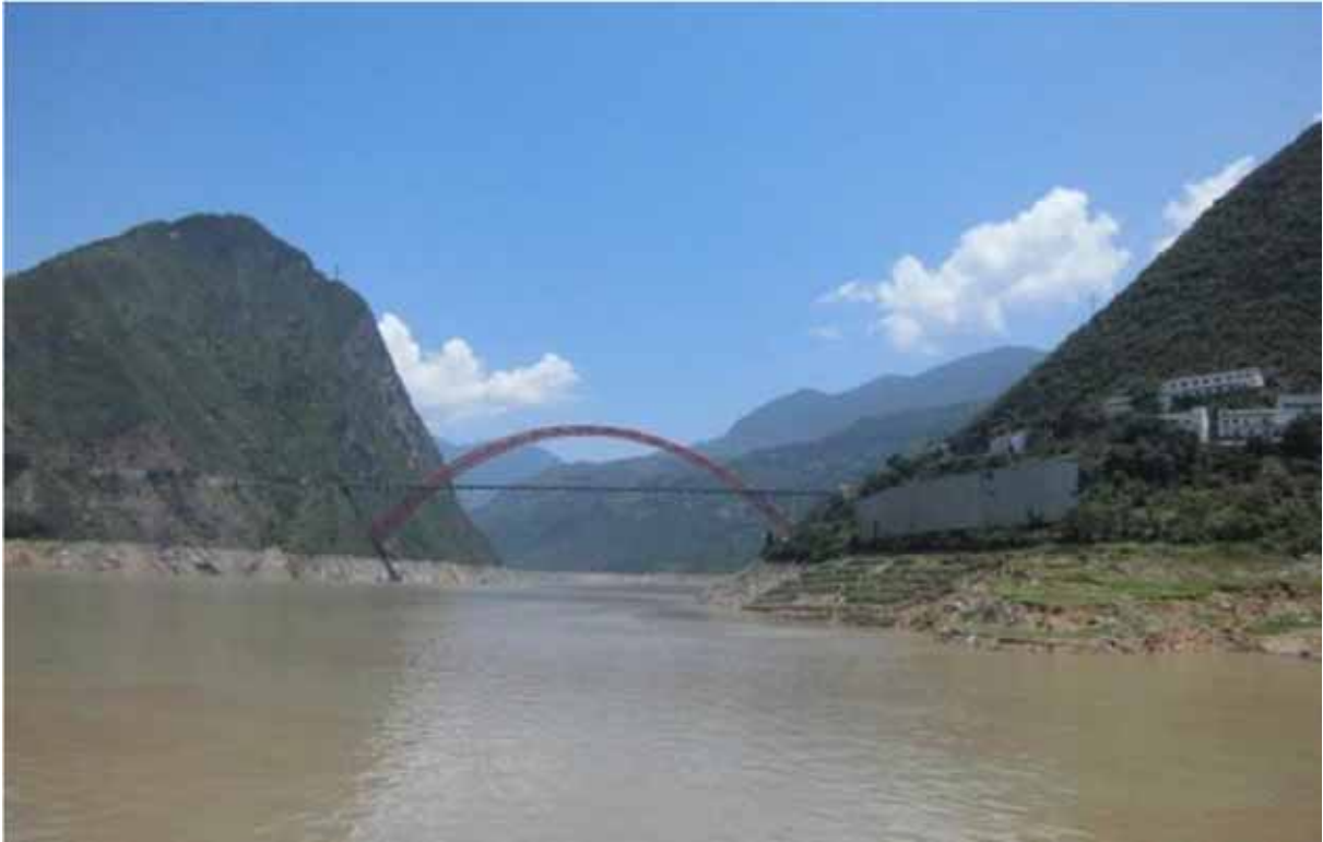
Wu Gorge Side Bridge
