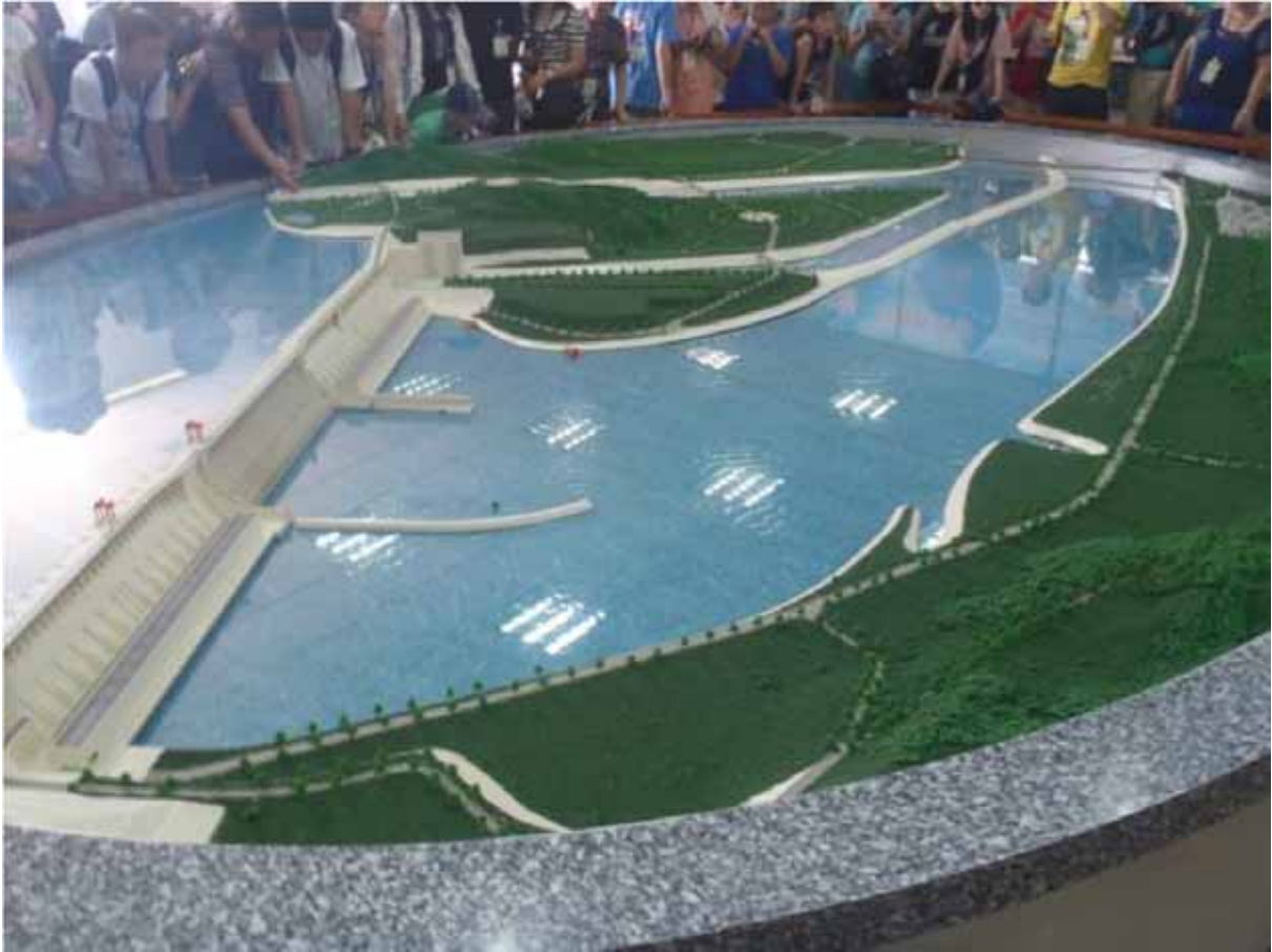
Three Gorges Dam model (14 north /12 south/ 6 underground/ 2 self-turbine generators)
