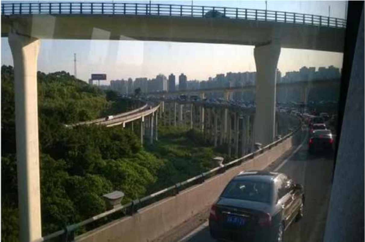
Chongqing City cloverleaf and elevated road traffic
