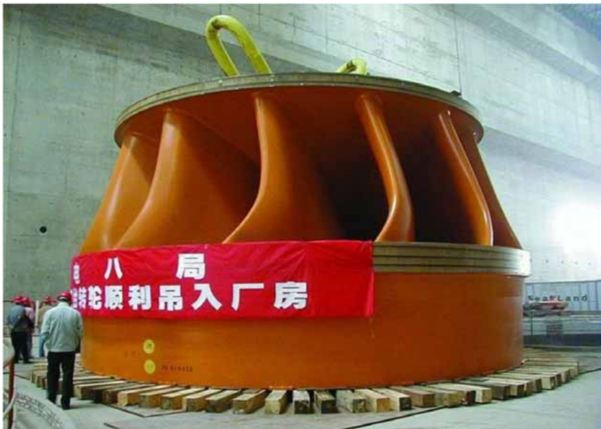
Francis turbine 10m wide and 9.8m tall
