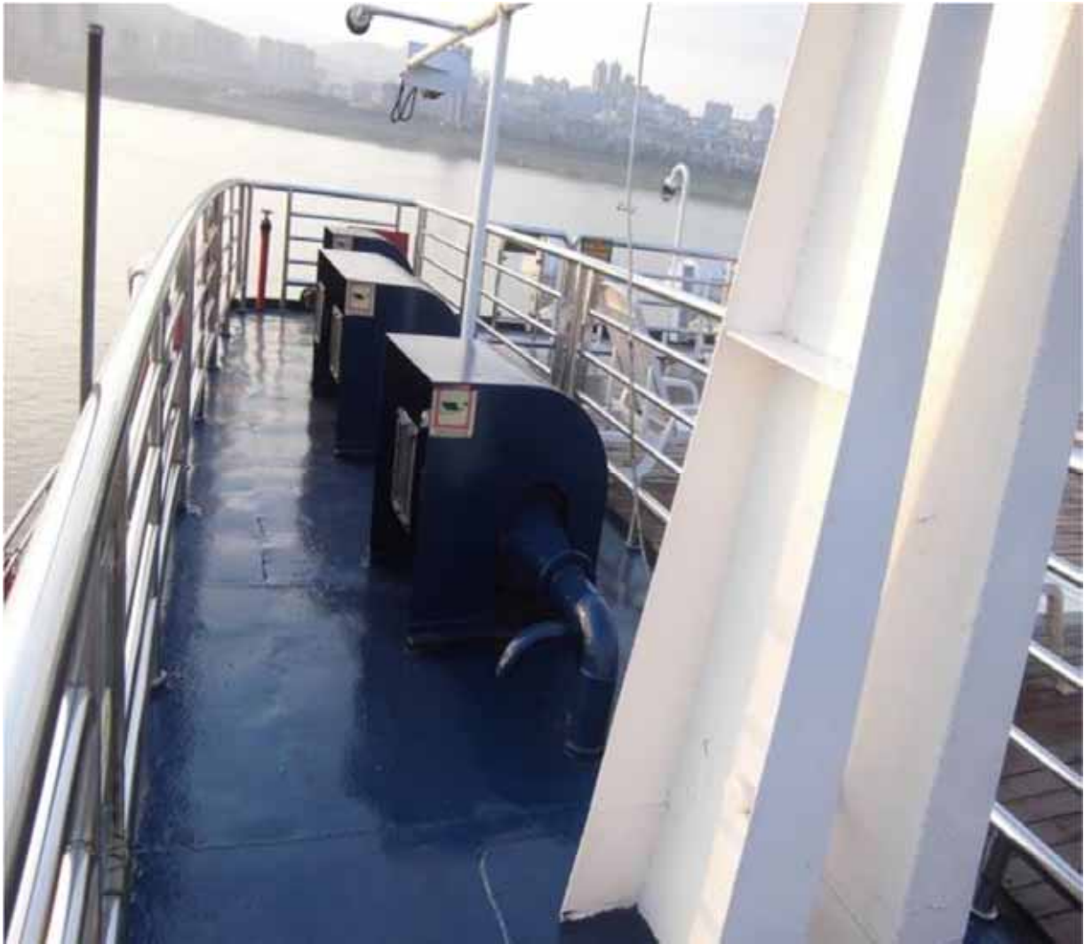
Deck6 aftermost ventilation dampers
