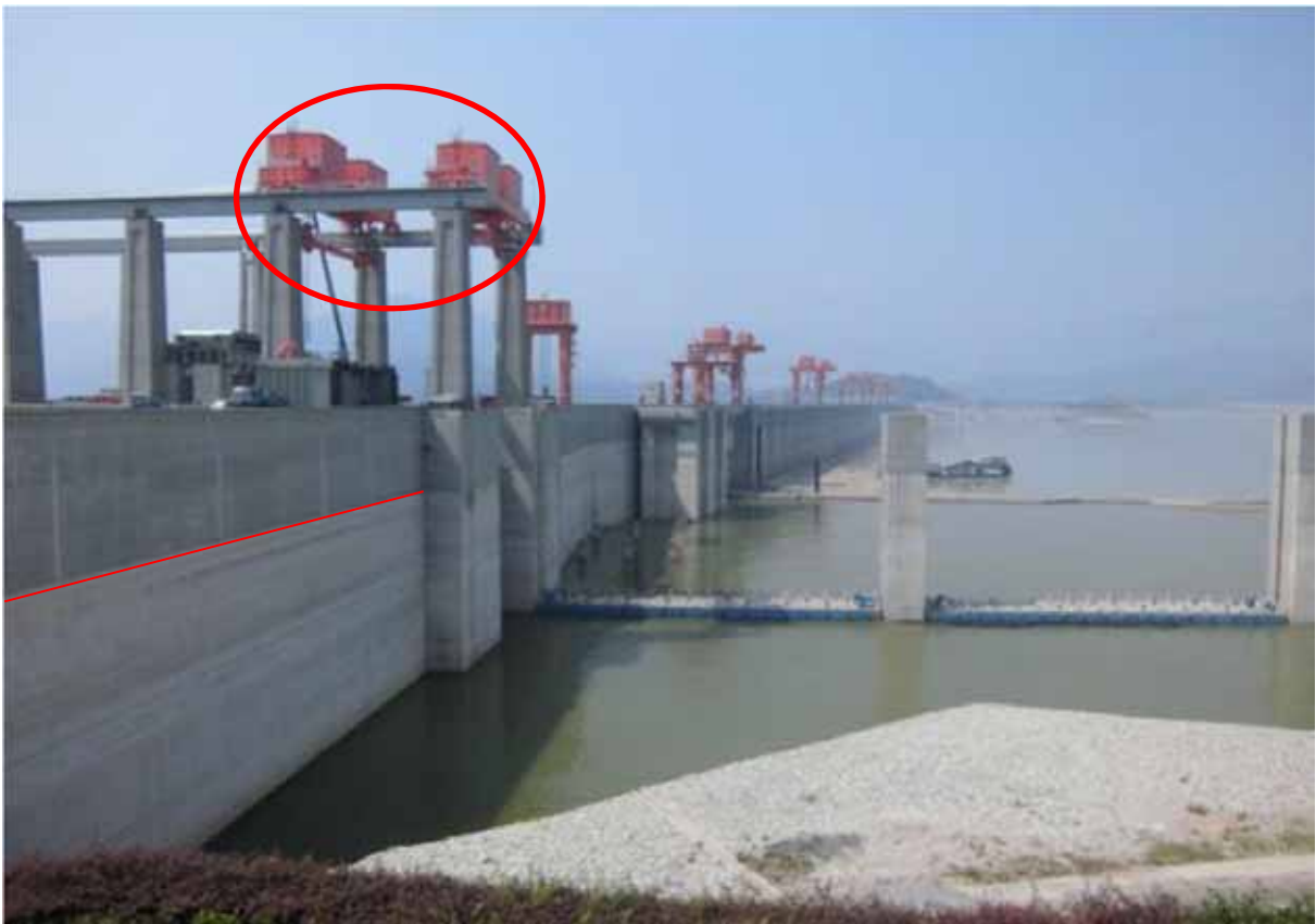
Three gorges dam with highest 175m water marks and four 195m towers for the ship lift
