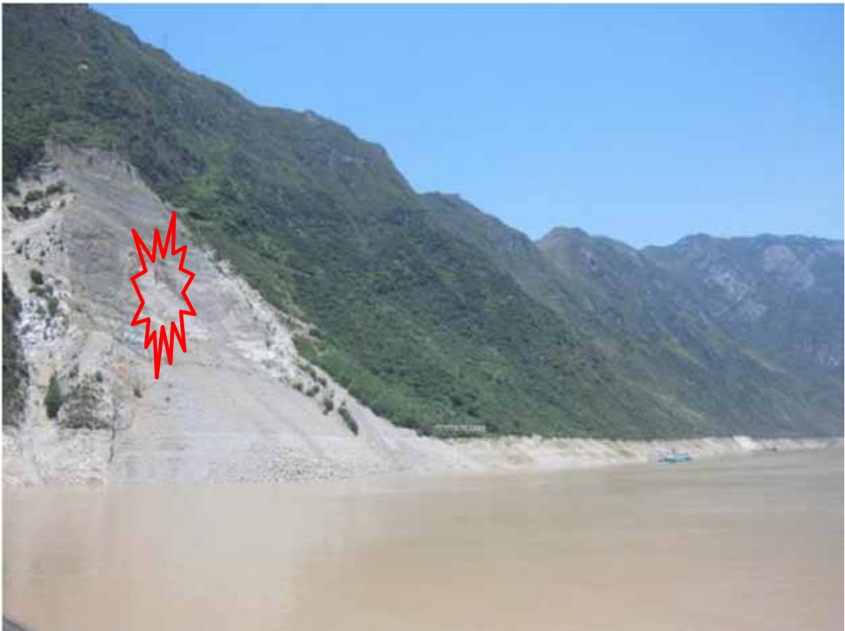
Yangtze River mountain slide repaired with highest water level marks
