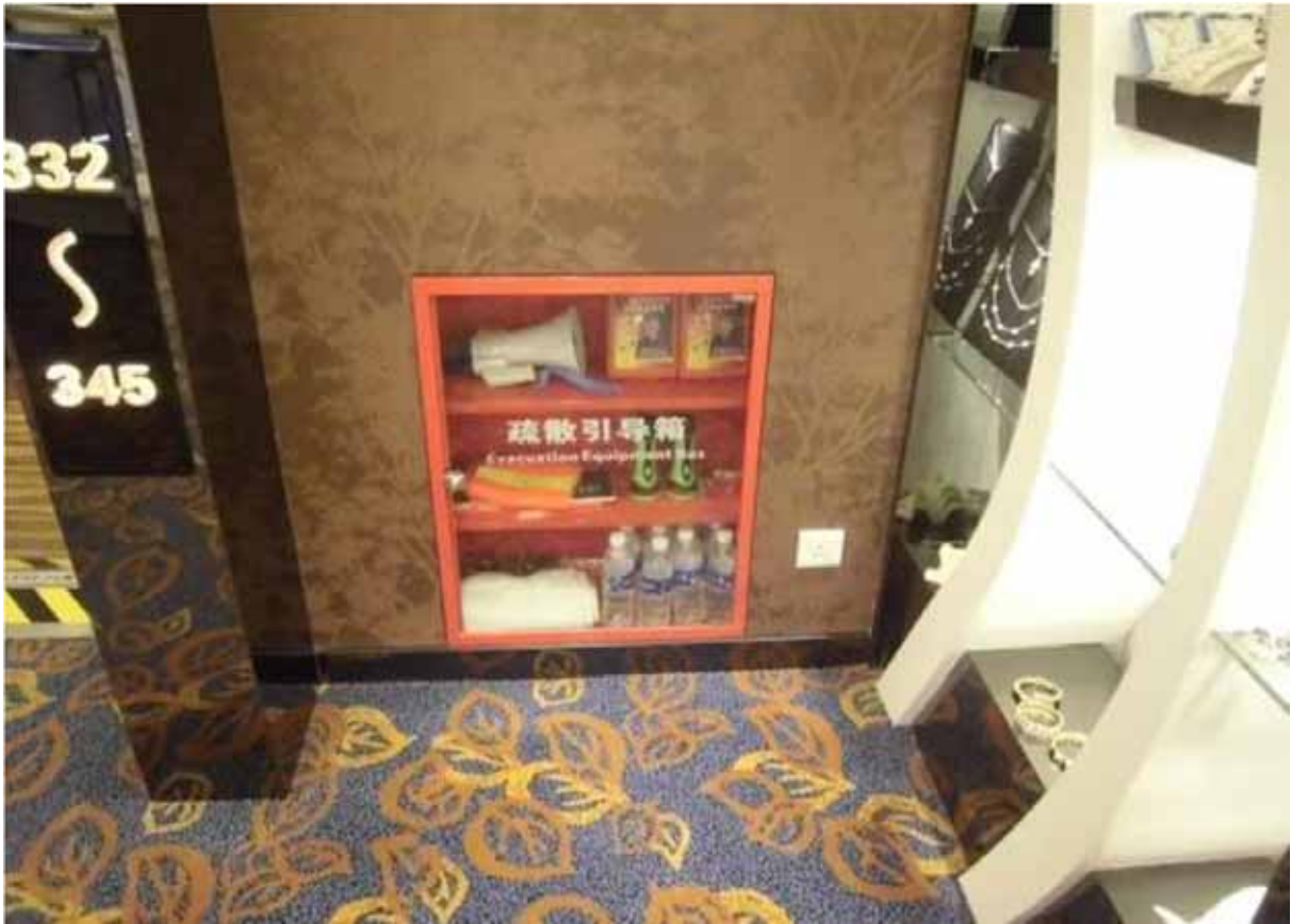
Evacuation equipment box
